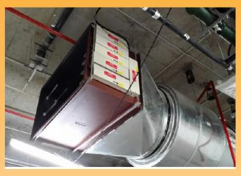
**Installation:** The DUO units are easy to install. Simply cut out the appropriate hole size on the duct and attached fixture with self tapping screws. Secure the lamps with the retainer plate and wire the input supply
