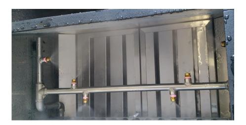
o Wipe and clean spray nozzles with warm water if spray nozzles are blocked use a sewing pin to unblock.
