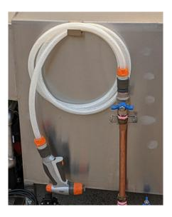
o Wash down and clean any large grease debris inside the unit and scrap any large debris and give the stainless filters a clean to remove any grease and oil via spray hose
